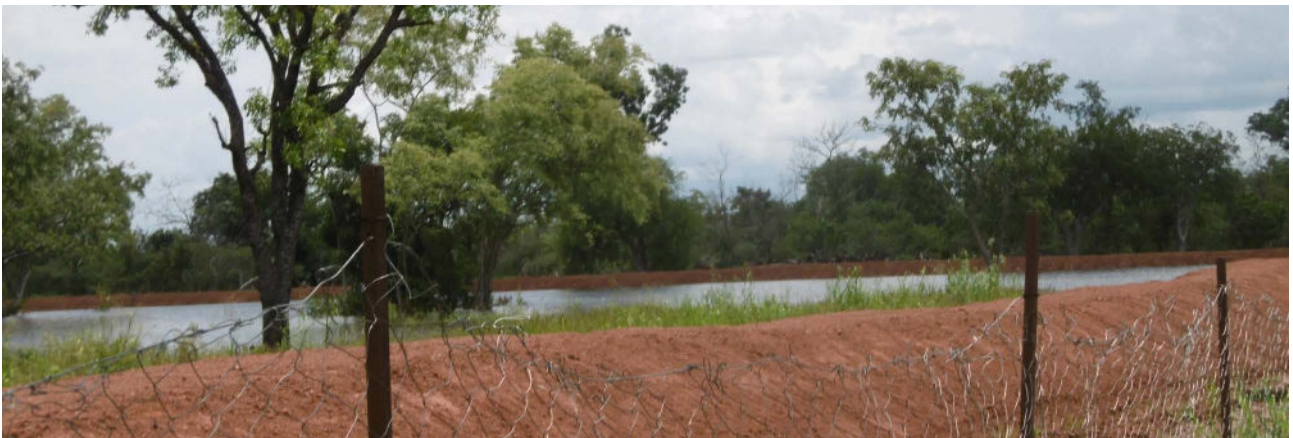
Wastewater basin, August 2018.
