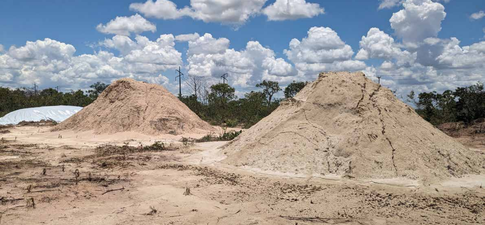
Piles of limestone to be spread on the cleared land. This limestone comes from mines and is used to reduce the acidity of the soil, which is too acidic in the region for soy crops. Photo taken during the field investigation in the Vale Do Urso farm (Barreiras).
